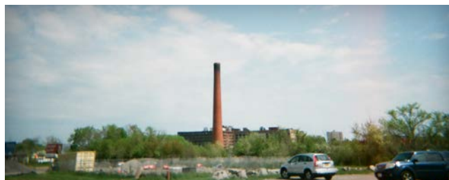
Old incinerator smokestack
