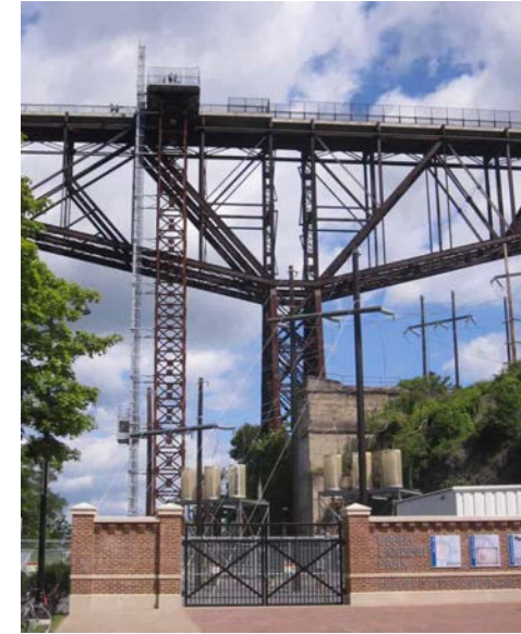
Walkway over the Hudson Elevator
