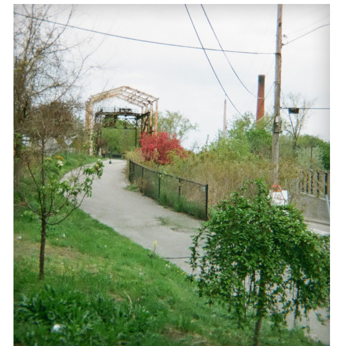
View of the old cooling tower
