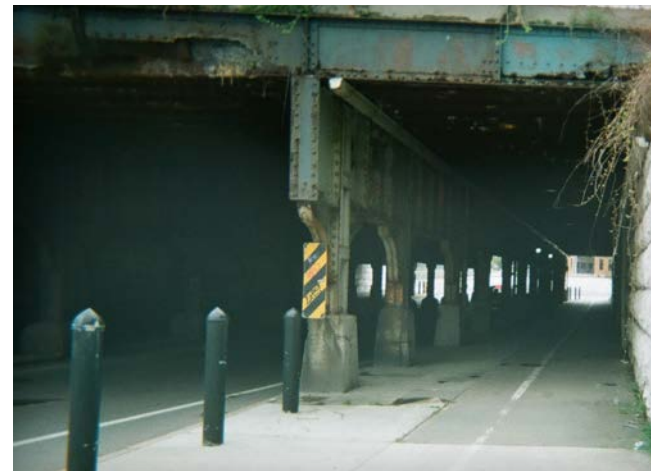
Pedestrian experience of St. Paul Street RR underpass (see 1.6)
